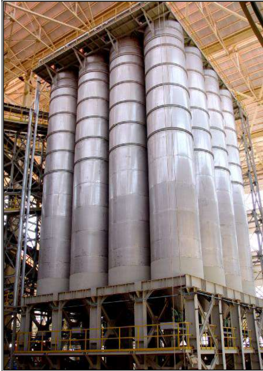
Silos of granol
